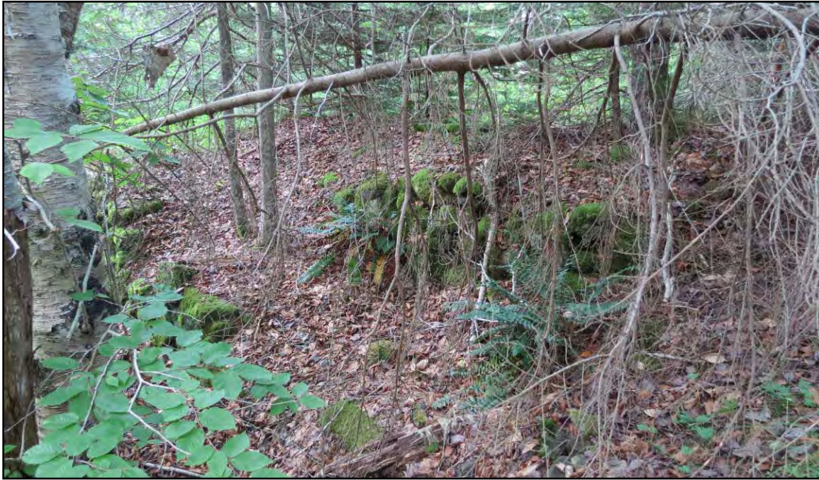
PLATE 15: Short section of off-set foundation wall at northwest corner of Henderson cellar; facing west. July 26, 2015.
